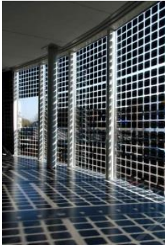
Building/Invisibly Integrated Photovoltaics (BIPV/IIPV)
